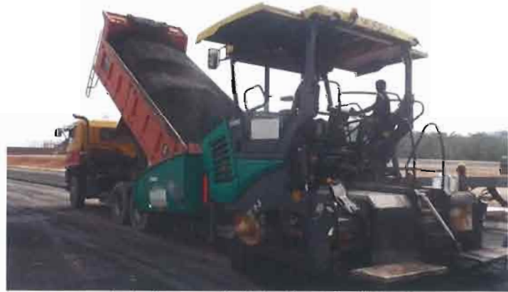
Asphalt paver set is laying the asphaltic layer
