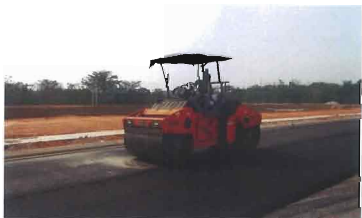
Compacting the asphaltic layer using a steel wheeled tandem roller
