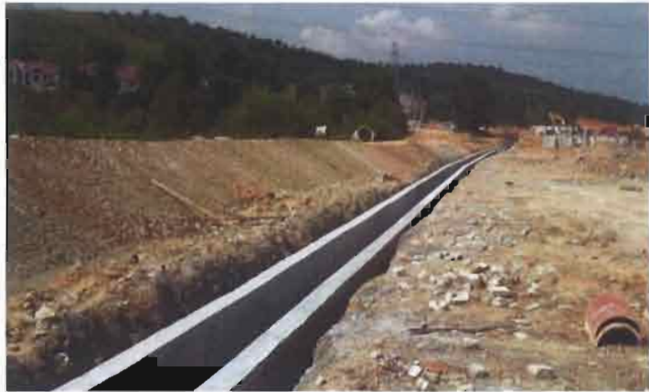
Drainage system installed prior to the construction of road
