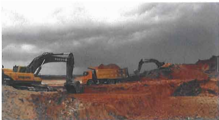
Crawler excavators loading soil into a dump truck
