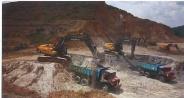
Step 1: Area with hard material is identified during excavation and fill
