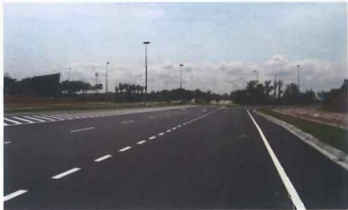
Completed roadway with pavement markings
