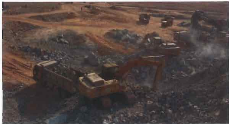
Step 4: Excavation of rocks after rock blasting
