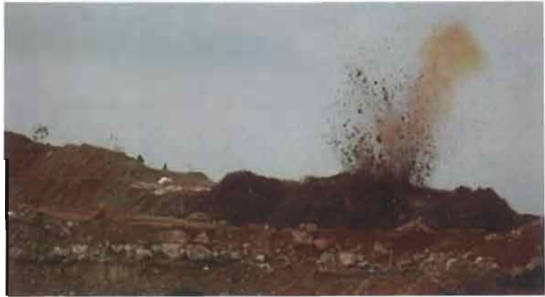
Step 3: Rock blasting
