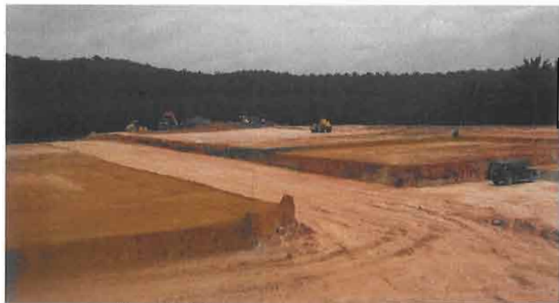
Compactor in the process of compacting fill material
