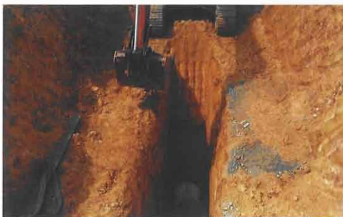
The reinforced concrete sewer pipes are laid down into the trench
