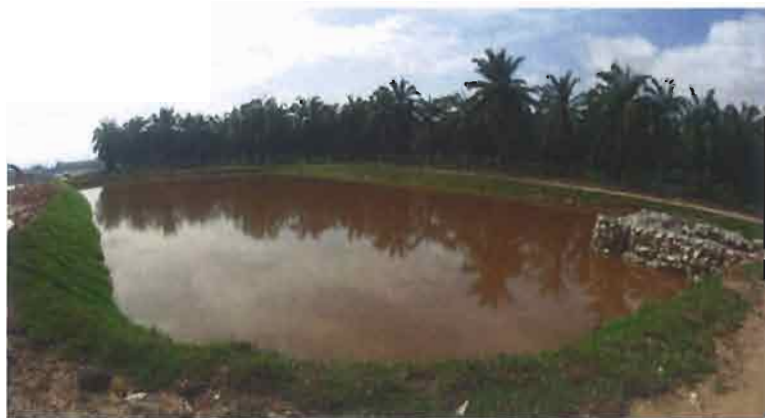
Sediment basin located within a project site
