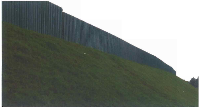
Turf being laid on a slope
