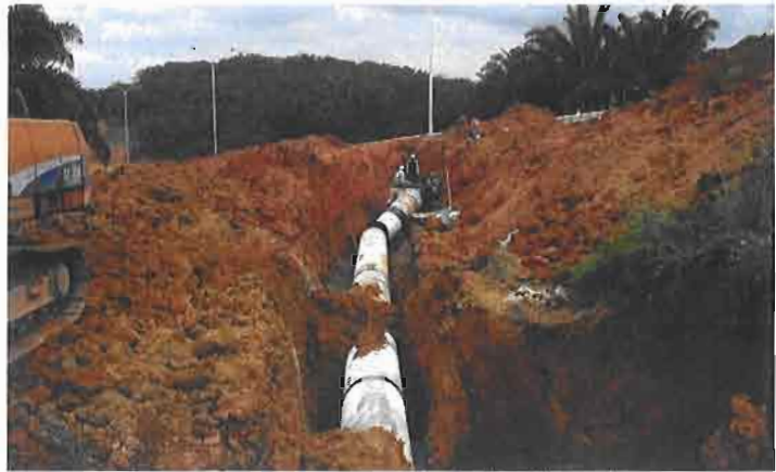
Welded pipes are laid and checked by the workers
