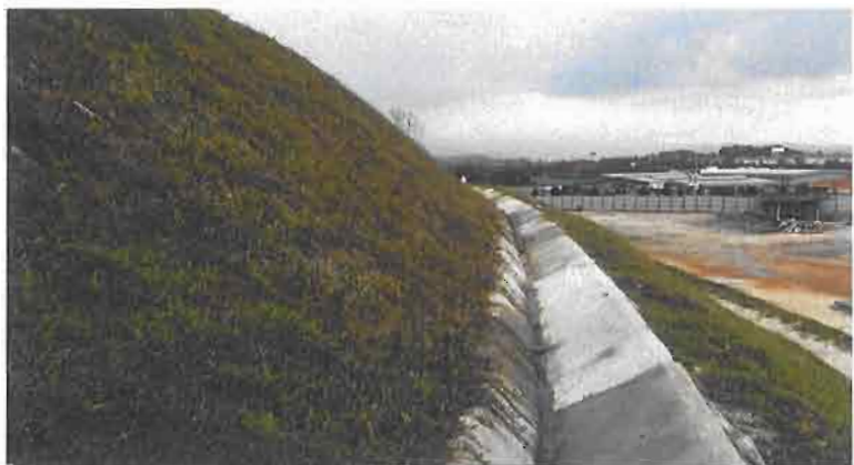
Berm drain being constructed on a slope
