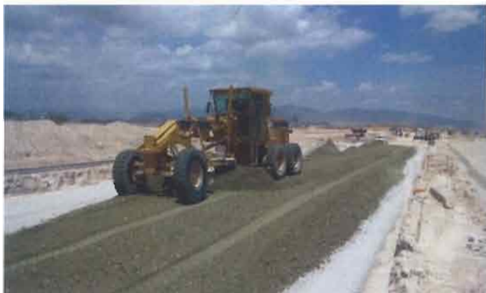
Levelling the road base with motor grader
